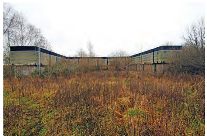
The air intakes and outlets on the roof of the bunker
